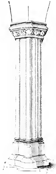
PIER: CLUSTERED PIER OF LATEST TYPE, WITH ONE CAPITAL FOR THE WHOLE. STOGUNBER, CHURCH OF S. MARY, SOMERSET: C. 1500.
